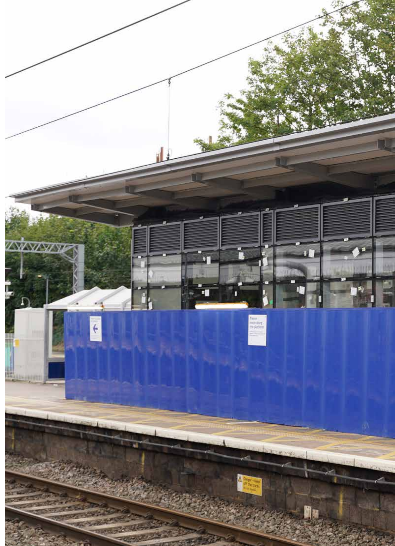
We are refurbishing 22 of our Elizabeth line surface stations
